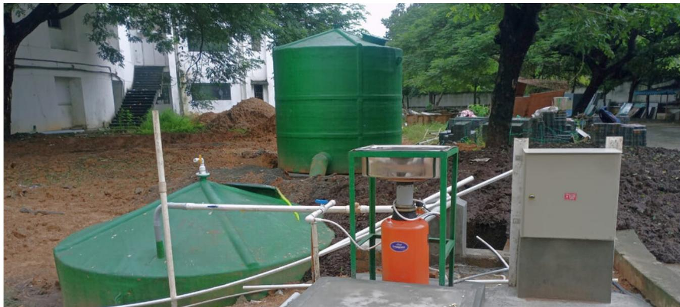
In a visionary move towards sustainable practices, Saveetha Institute of Medical and Technical Science in Kanchipuram has recently embraced a green initiative by installing a cutting-edge Green Connect Biogas Plant. The installation, designed to process 500 kg of food waste daily from the institute's canteen, has become a beacon of environmentally conscious energy solutions.
